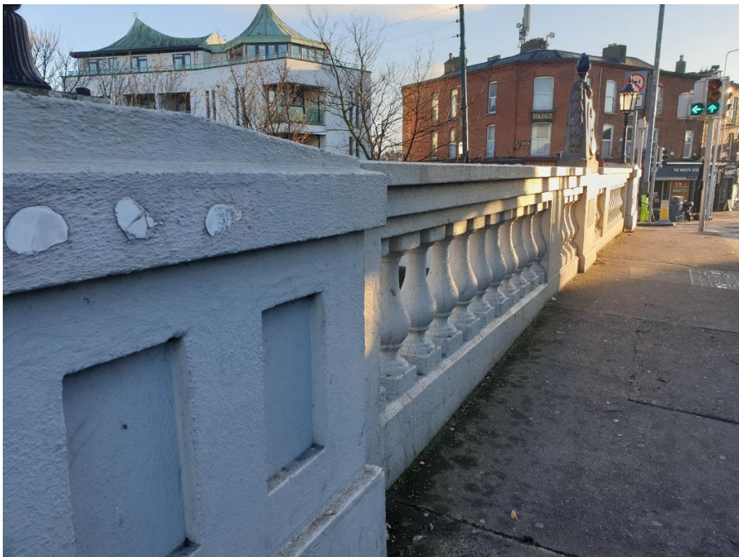
Footpath and parapet of Robert Emmet bridge
