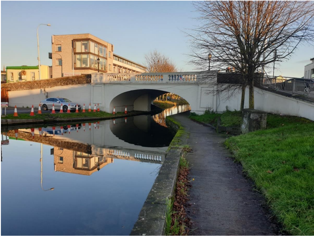
Existing Robert Emmet Bridge – looking from the West side where Kimmage 01A will be located
