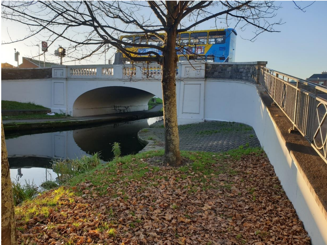
Existing Robert Emmet Bridge – looking from the East side where Kimmage 01B will be located
